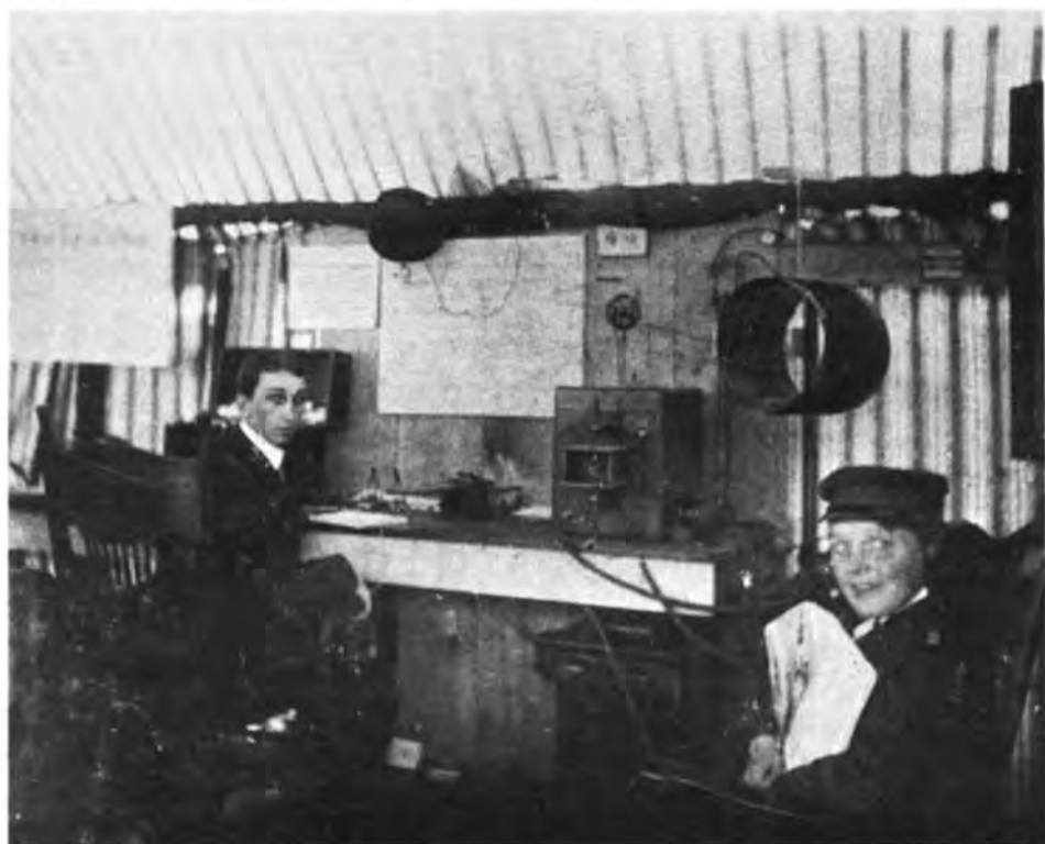
Interior view of the DeForest wireless station on exhibit during August and September 1903 at the Canadian National Exhibition, Toronto, one of the first wireless telegraph stations in Canada.
